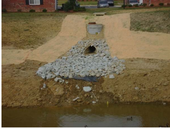
Erosion control measures at pond inlet.
