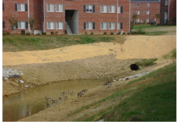
Pond bank stabilized with erosion control matting.
