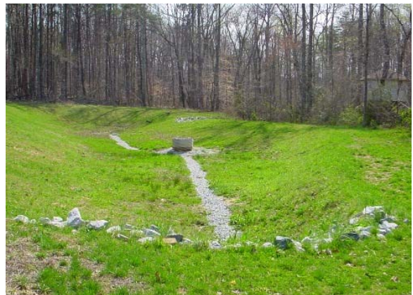
Dry detention with gravel filter strip.
