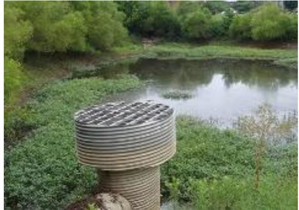
Non-compliant pond with failed riser.
