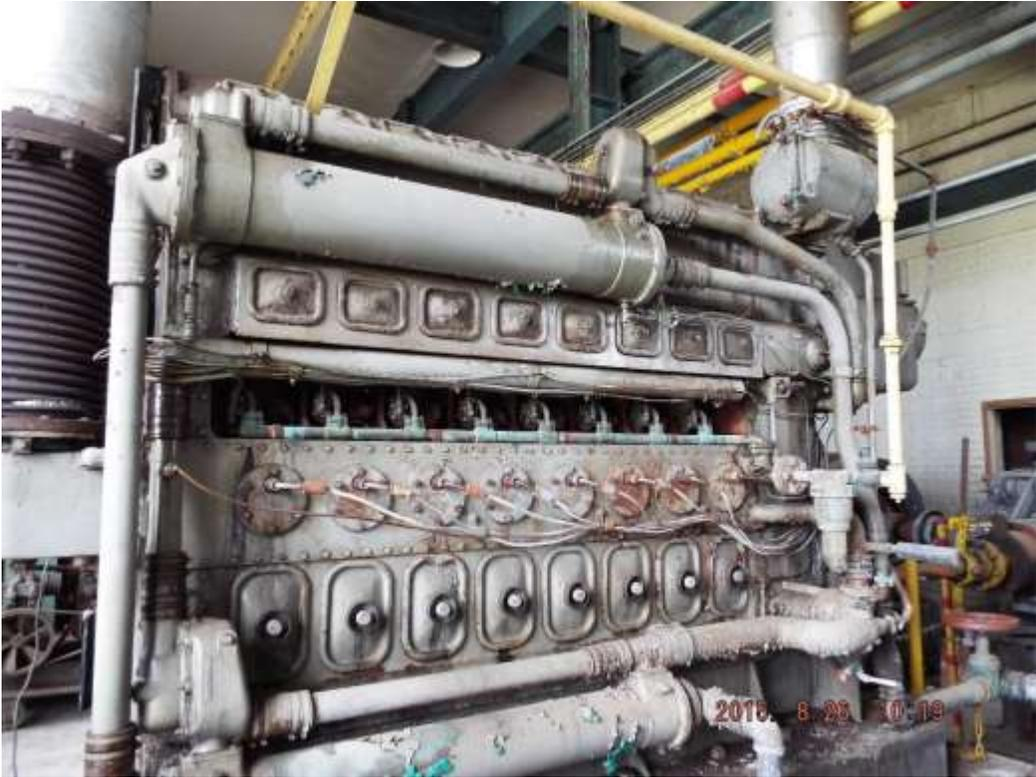
Diesel engine on 1st floor used in the past for emergency backup power
